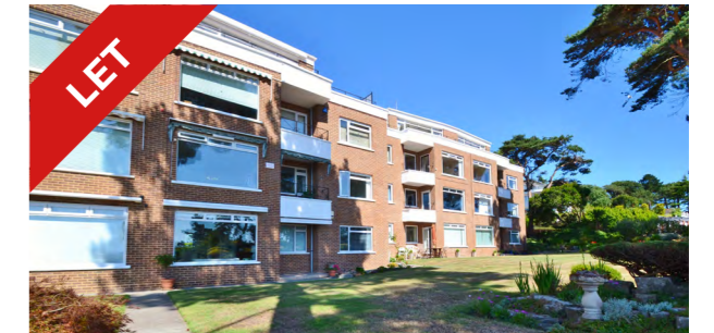
Waters Edge: 2 bedroom, 2 bath ground floor unfurnished apartment in Canford Cliffs with stunning harbour views
